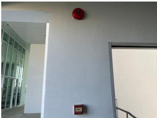
Manual Station and Alarm Bell
